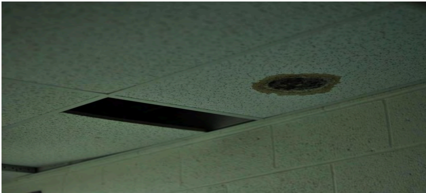
Missing ceiling tiles and unknown substance stains are in addition to potential health hazards in Welte Theatre's basement.
