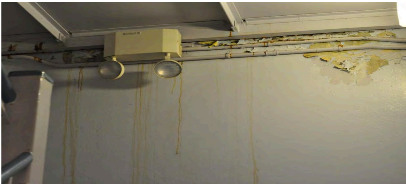
Welte Theatre experiences leaking issues within their basement, amongst several other problems.
