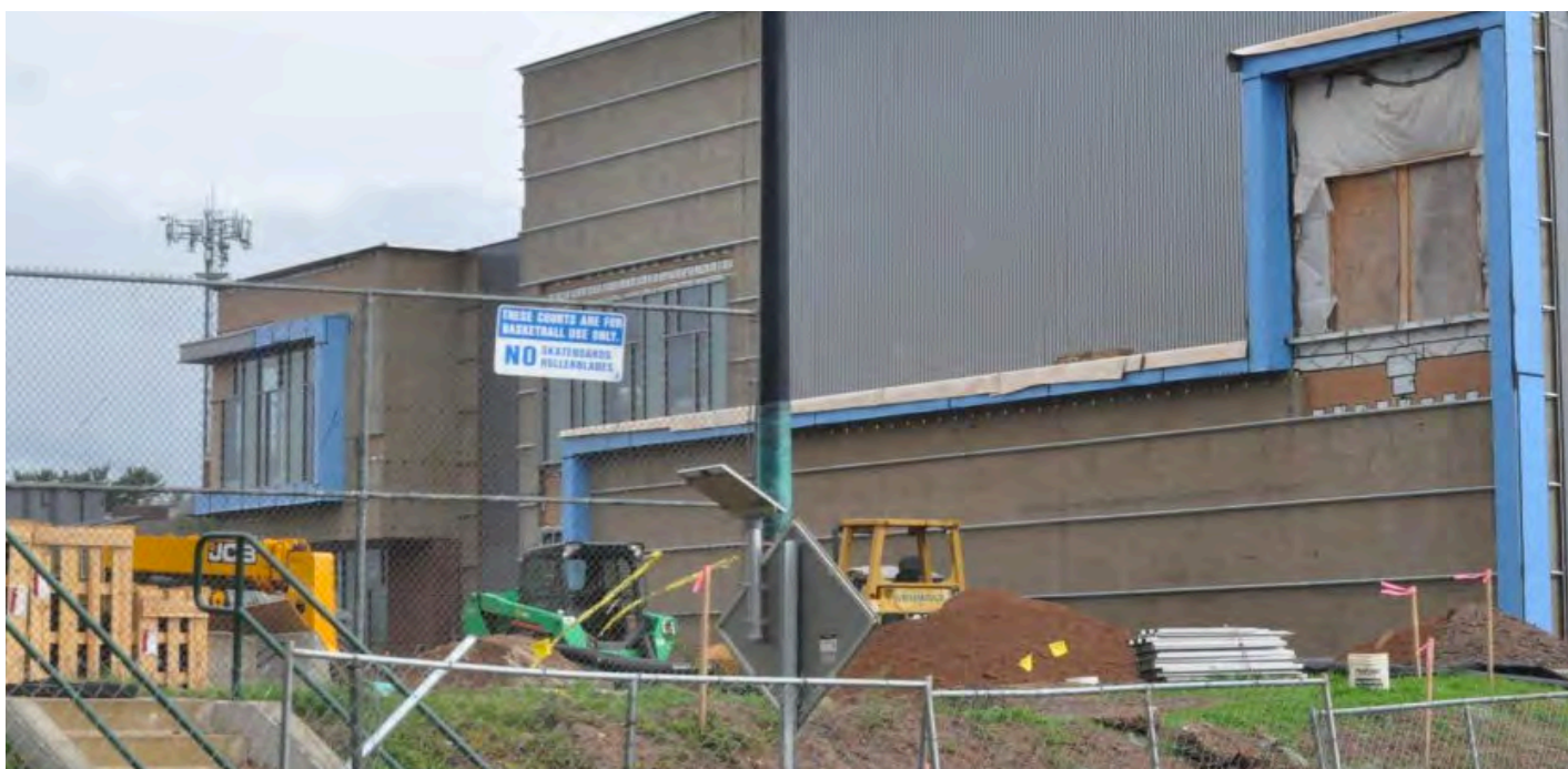
Construction is still underway for the Recreation Center.
