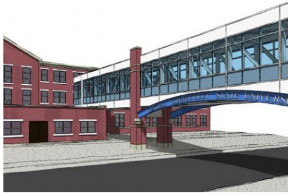
The parking lot will have a glass walkway connecting it with Willard-Diloreto
