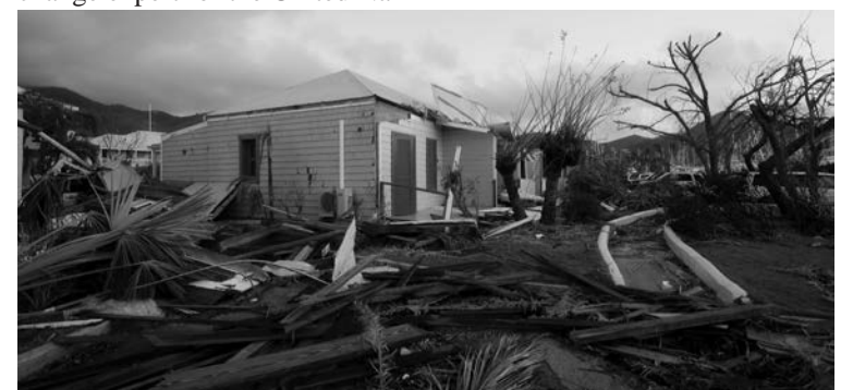
Damage to buildings from Hurricane Irma, Nanny Cay, Tortola, Sept. 17, 2017. Photo courtesy of Flickr/DFID
