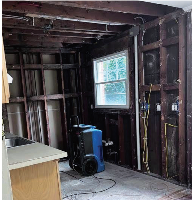
Inside of the kitchen in the apartment on Savin Ct., mid-construction, West Haven, Oct. 7, 2022 Photo courtesy of Charger Bulletin/Melanie Kirtman.
