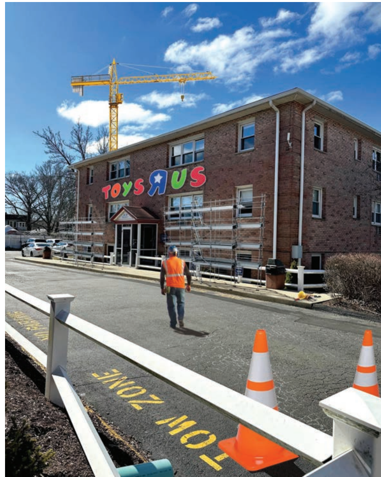
Construction commences, West Haven. Graphic courtesy of Charger Bulletin/Jacey Ferraro.
