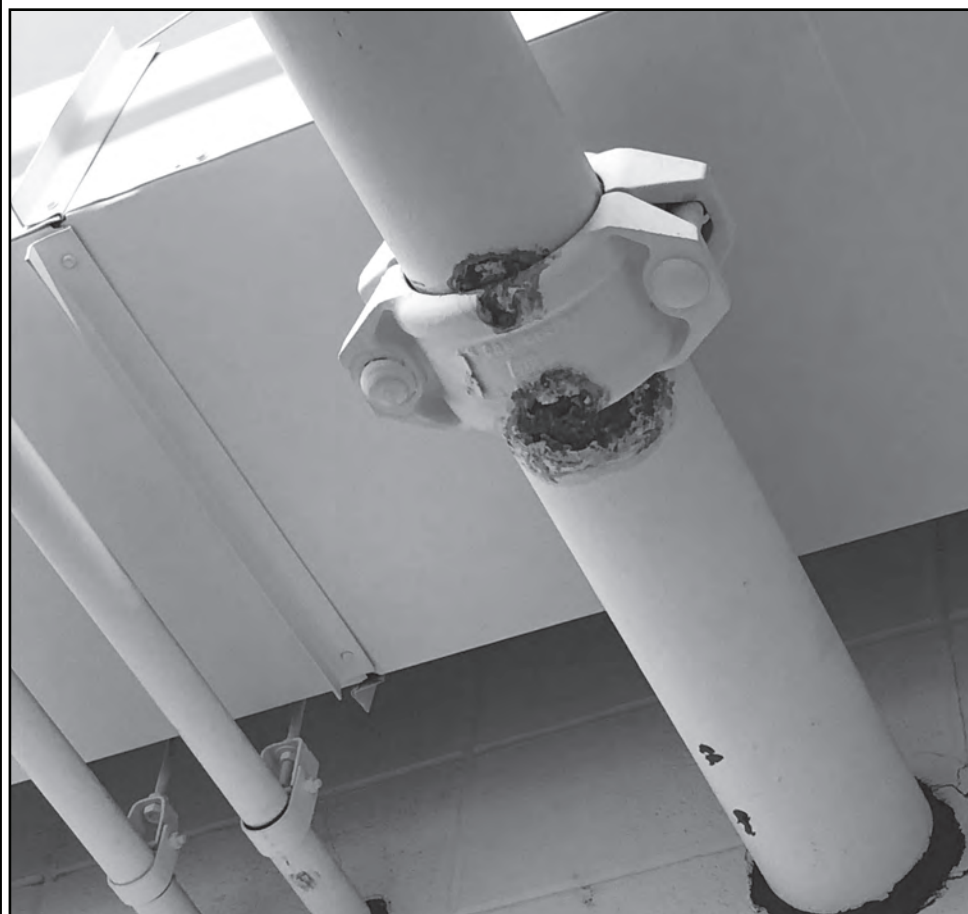
MOLD INFESTATION A mold covered pipe found in the basement of Westhill.
