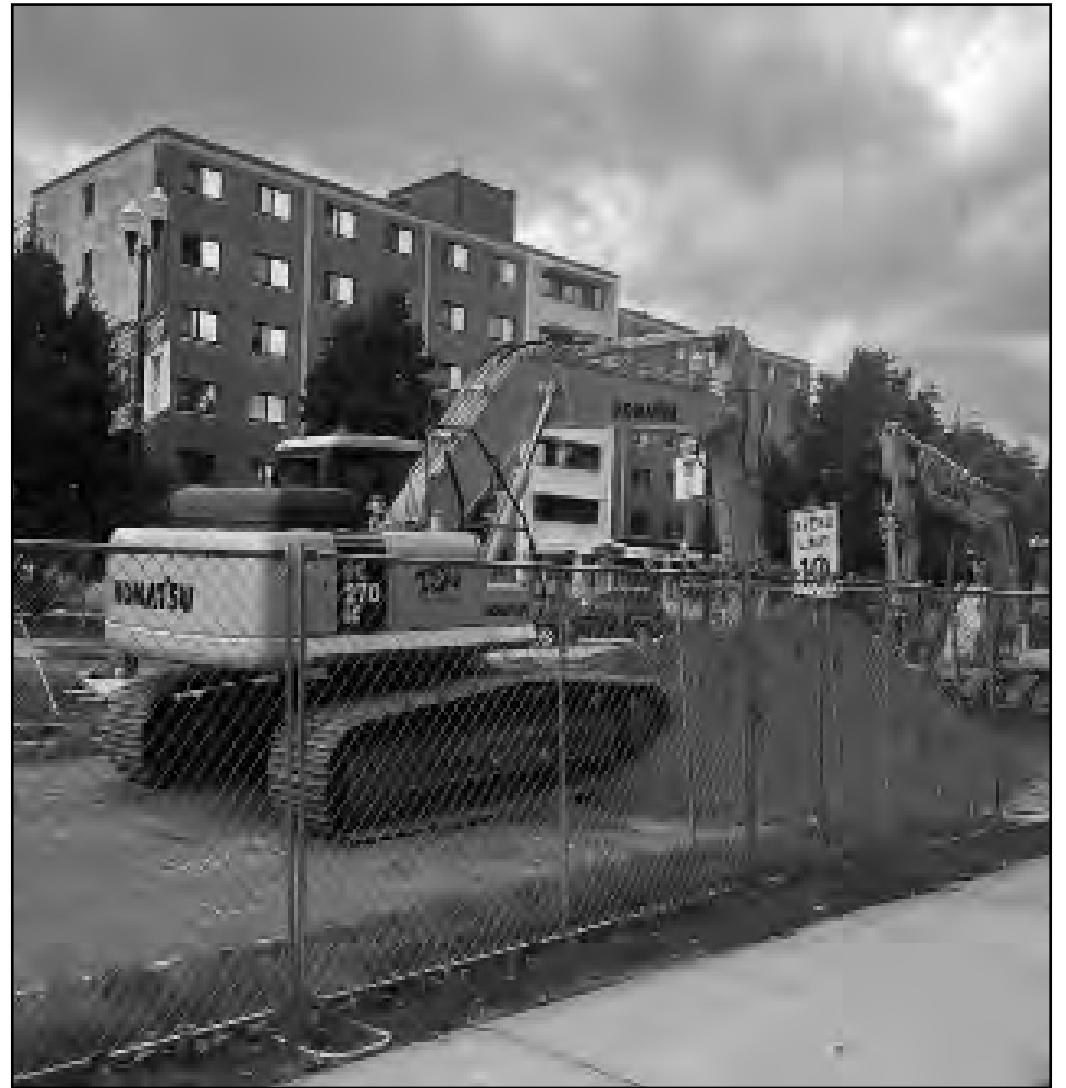
Construction project located behind Chase Hall on Aug. 6.
